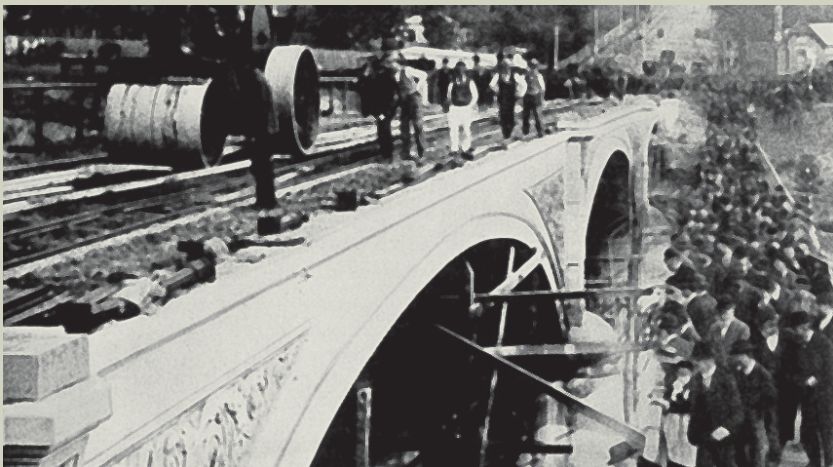
Anderson Street bridge, designed by Monash, during construction.
