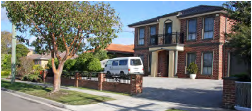
Typical increase to site coverage in residential land use in the City of Monash
