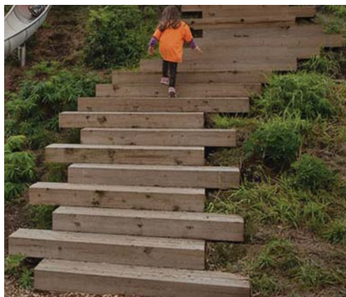
timber steps in side of slope
