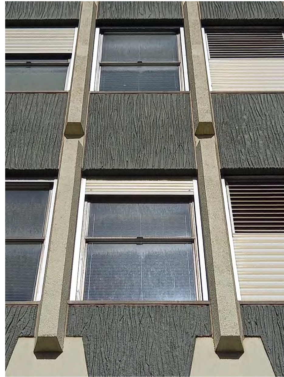
WINDOW TYPE A - EXISTING CONDITION PHOTO
