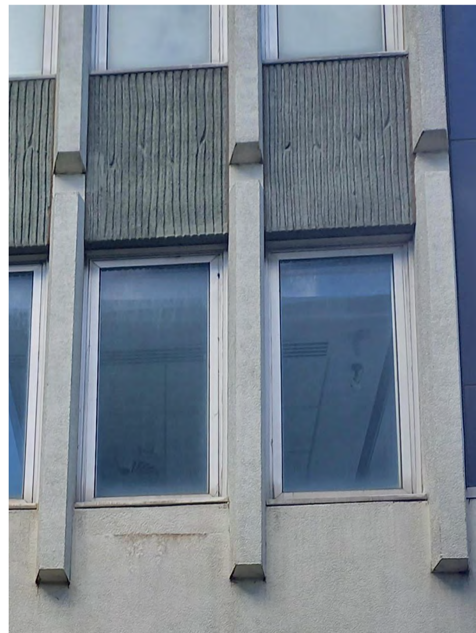
WINDOW TYPE H - EXISTING CONDITION PHOTO
