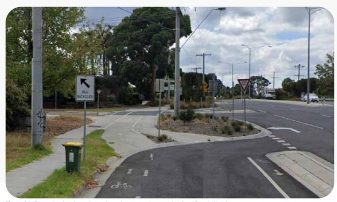
Figure 24. Example of cycle path cut through at street intersection Stud Road, Wantirna
