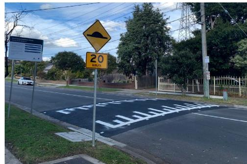
The road humps would be full width and lower in height. The modified flat topped road hump is lower than a standard hump (75mm high instead of 100mm). It provides a smoother drive and reduces noise, while still addressing speed concerns.
