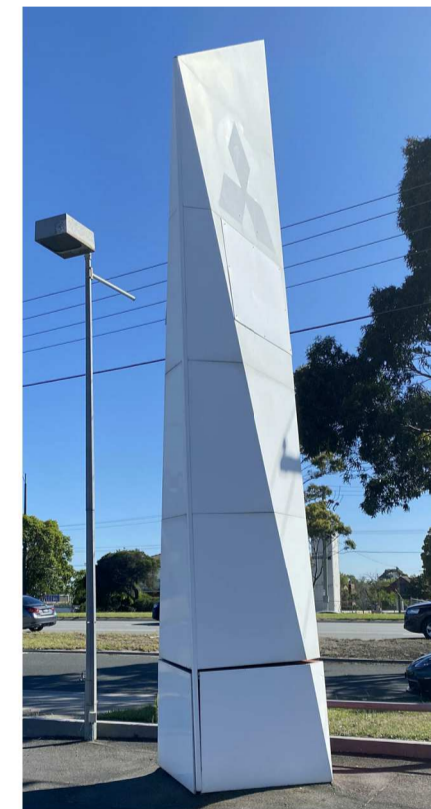
EXISTING SITE PHOTO
