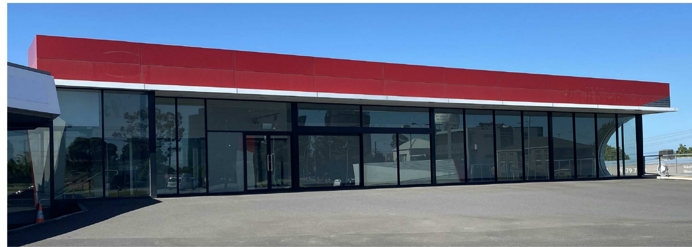
EXISTING SITE PHOTO
