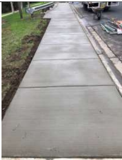
Wellington Road, Mulgrave (Freeway Overpass)
