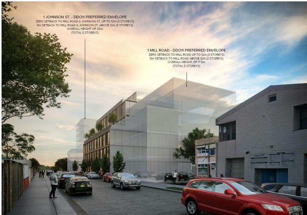
*3D perspective showing approved building form from Mill Road, with proposed building envelope shaded*
