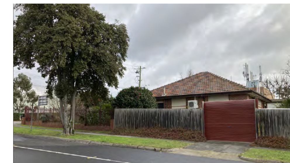
VIEW 05 - SUBJECT SITE FROM EAST
