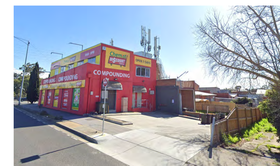
VIEW 14 - NO 545 WARRIGAL ROAD 2 STOREY BRICK COMMERCIAL
