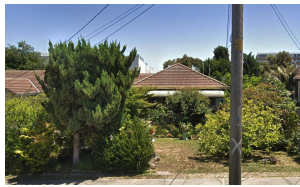
▲ 01 NO.21 TERRIGAL ST CHADSTONE 1 SINGLE STOREY BRICK DWELLING/ TILE ROOFING
