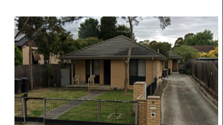
▲ 08 NO.30 COLLINS ST CHADSTONE 1 SINGLE STOREY BRICK DWELLING/ TILE ROOFING/METAL FENCE
