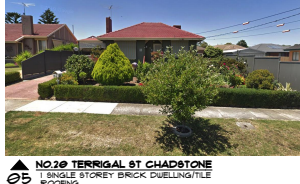
▲ 05 NO.29 TERRIGAL ST CHADSTONE 1 SINGLE STOREY BRICK DWELLING/TILE ROOFING
