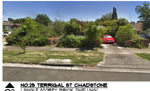
▲ 03 NO.25 TERRIGAL ST CHADSTONE 1 SINGLE STOREY BRICK DWELLING/ TILE ROOFING
