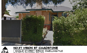
▲ 04 NO.31 VISION ST CHADSTONE 1 SINGLE STOREY BRICK DWELLING/TILE ROOFING/TIMBER FENCE
