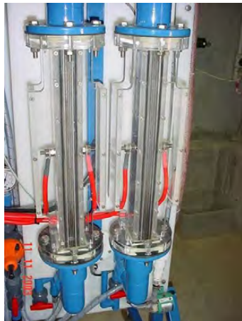
Sodium hypochlorite generation cells.
