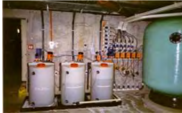
Typical sodium hypochlorite storage and dosing facilities.
