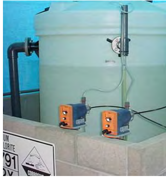
Typical sodium hypochlorite storage and dosing facilities.
