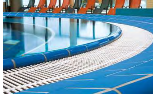
Weisbaden Wet Deck Pool Edge.
