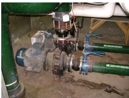
Typical pool pump configuration with filter cell multi-port valve.
