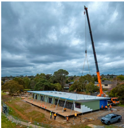
Built using a modular construction method, the new pavilion at Brandon Park Reserve is now open for business.
