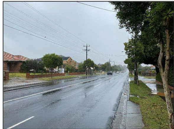
Figure 5: Clayton Road – View South
