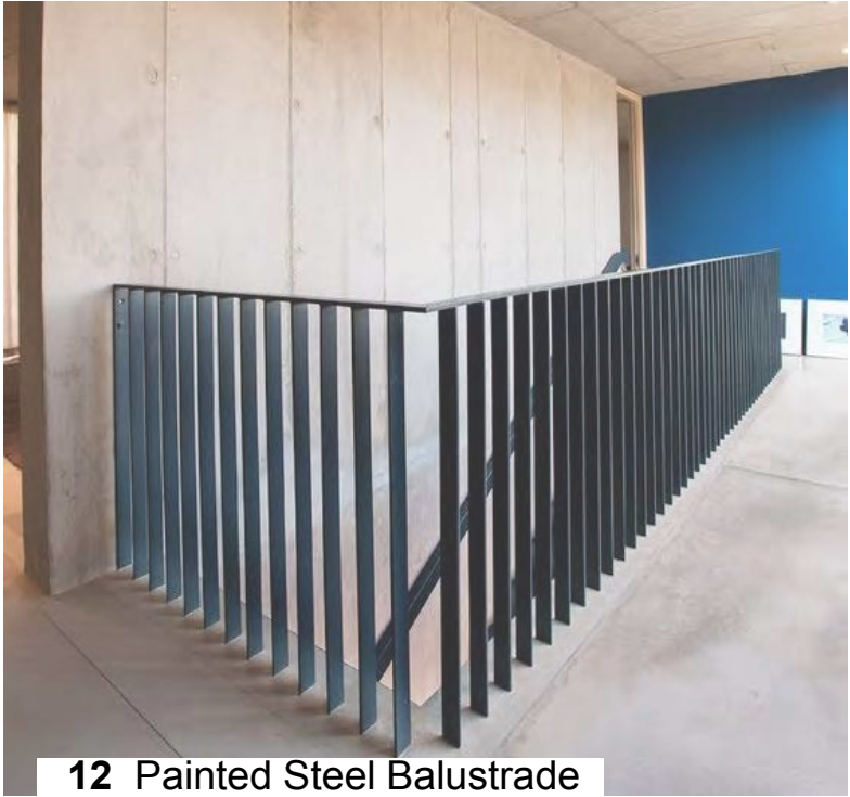
12 Painted Steel Balustrade
