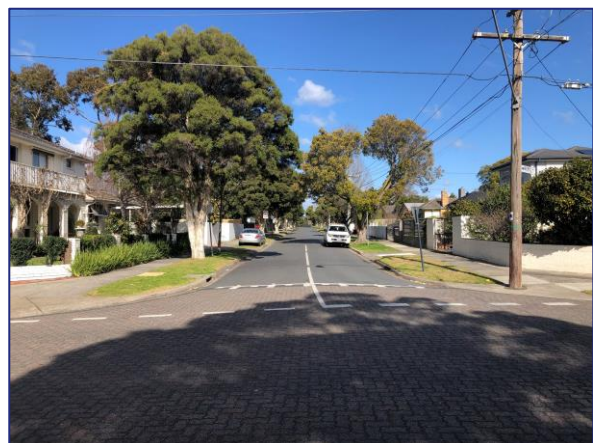
Figure 10: Bakers Road - view south
