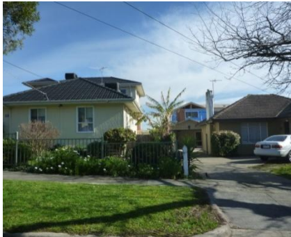
Discreet extensions and modifications located behind dwelling
