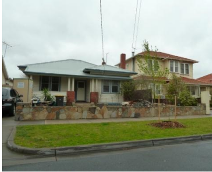
Second storey "pop ups"
