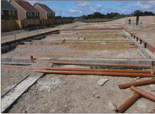
Void during construction
