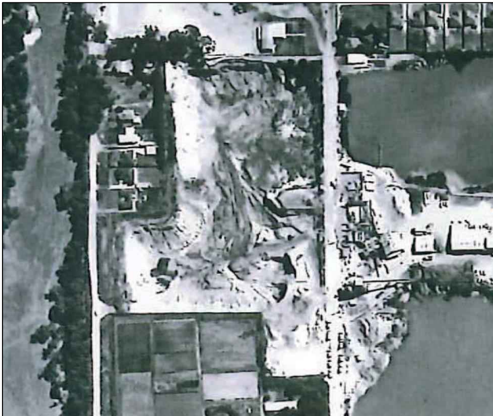
Plate 1 - Aerial photograph of Zone 1 from October 1970
