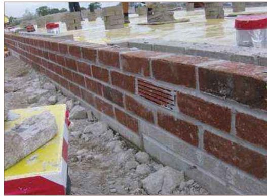
Finished gas membrane on plot 37
