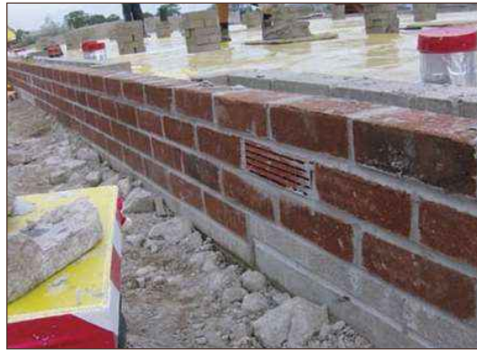
Finished gas membrane on plot 37
