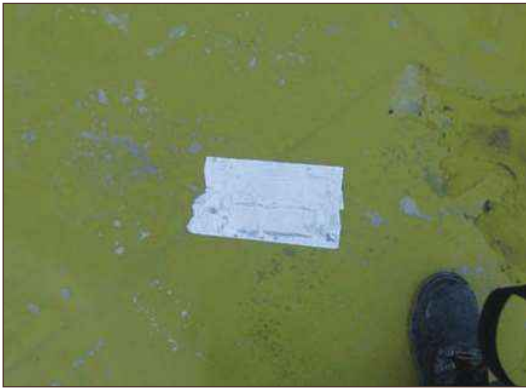
Finished gas membrane on plot 36
