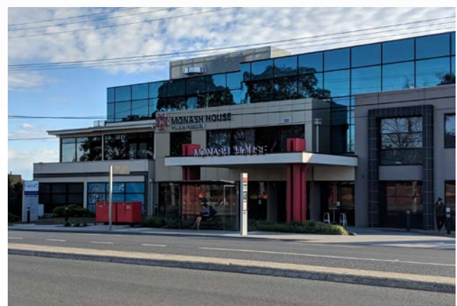
Image 4. Monash House Private Hospital
