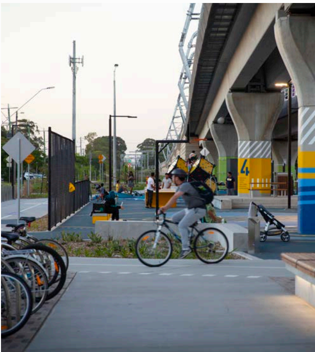
Image 19. Upgraded shared path infrastructure
