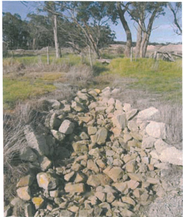
Rock lined discharge point to prevent erosion.
