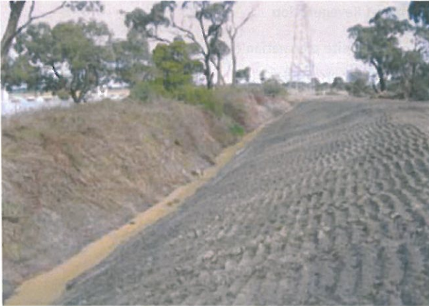
Reclaimed quarry face, cross ripped and hydroseeded.
