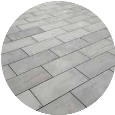
PAVING - TYPE 02 SEGMENTAL LARGE FORMAT PAVEMENT
