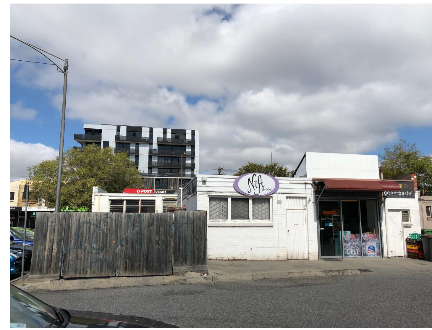
SITE REAR EXISTING CONDITION E
