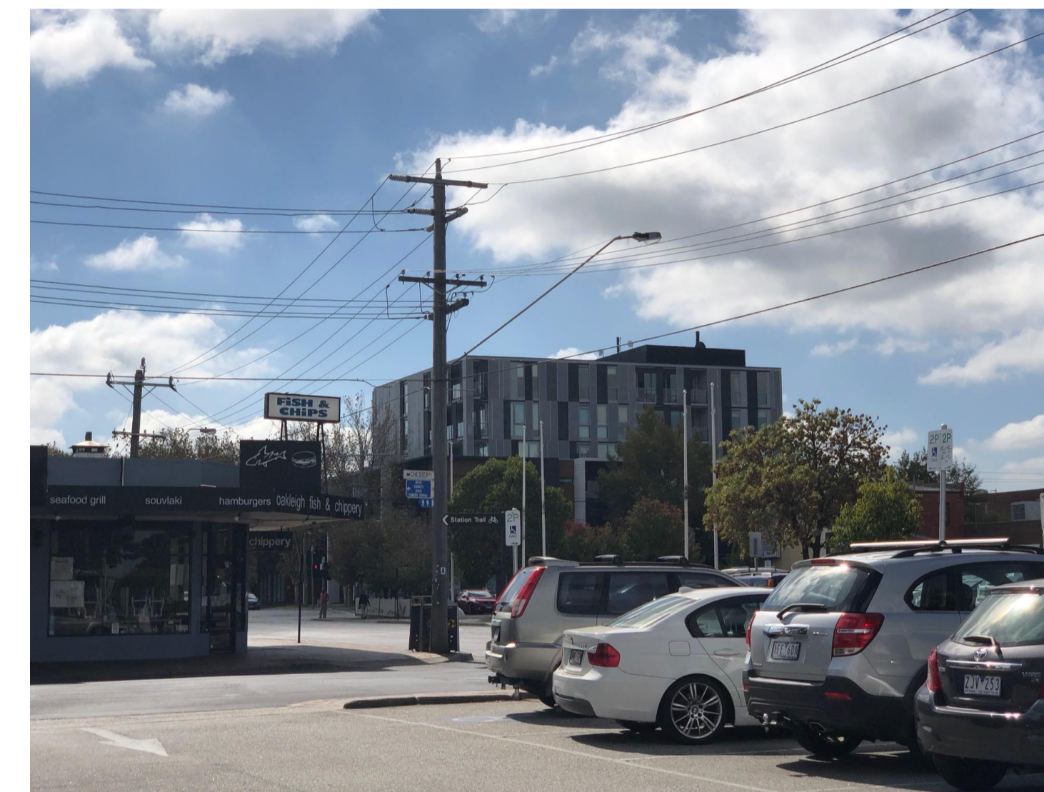
EXISTING 6-STOREY APARTMENT BUILDING G
