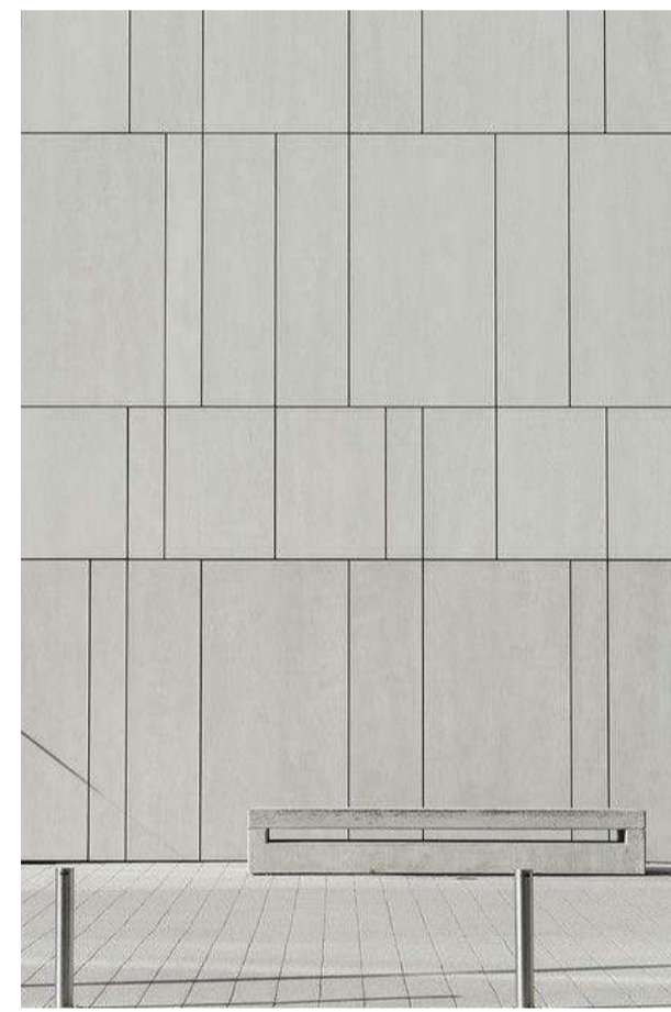
CN01 PRECAST CONCRETE- OFF WHITE
