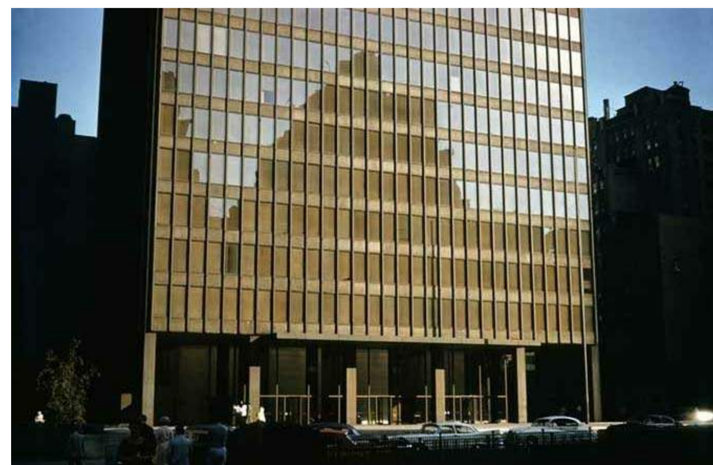
GL04 BRONZE GLAZING IN ALUMINIUM FRAMES. ANODISED FINISH - SATIN LIGHT BRONZE
