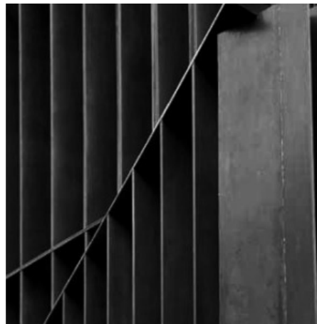
MT01: METAL FENCE/ SLATS POWDERCOAT FINISH COLOUR: DARK GREY DULUX "MONUMENT" OR APPROVED SIMILAR
