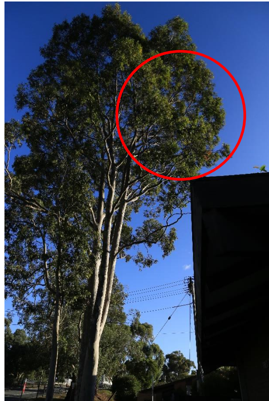
Figure 5.6. Canopy branches extending over roof of church building in tree 2.
