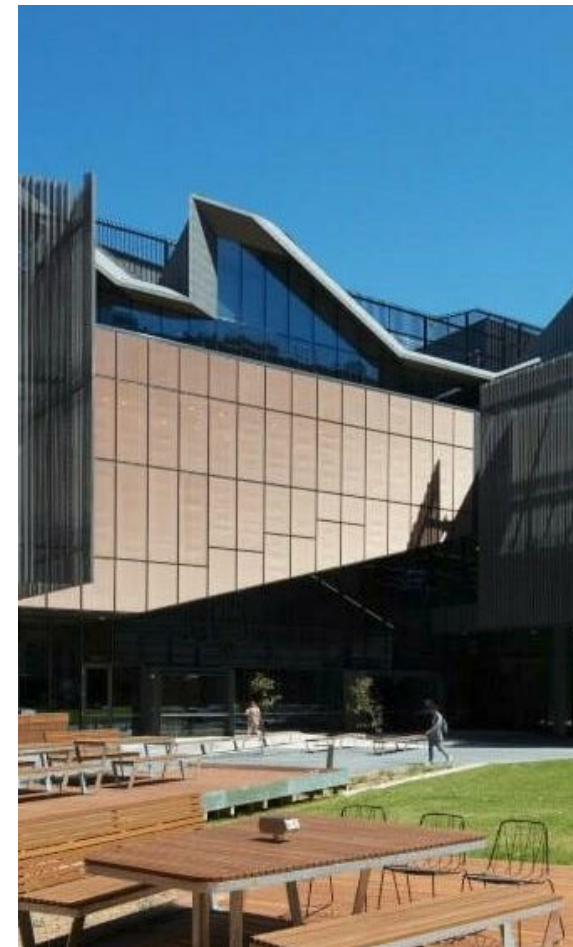
MONASH UNIVERSITY, CLAYTON CAMPUS GATEWAY BUILDING
